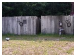
③ 鷺林寺南配水槽
